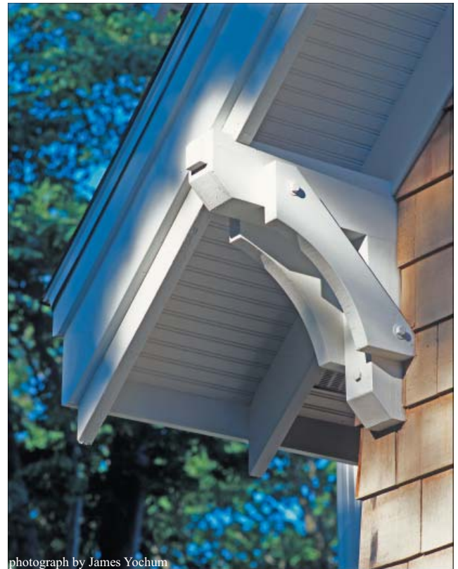
detail of roof brackets
