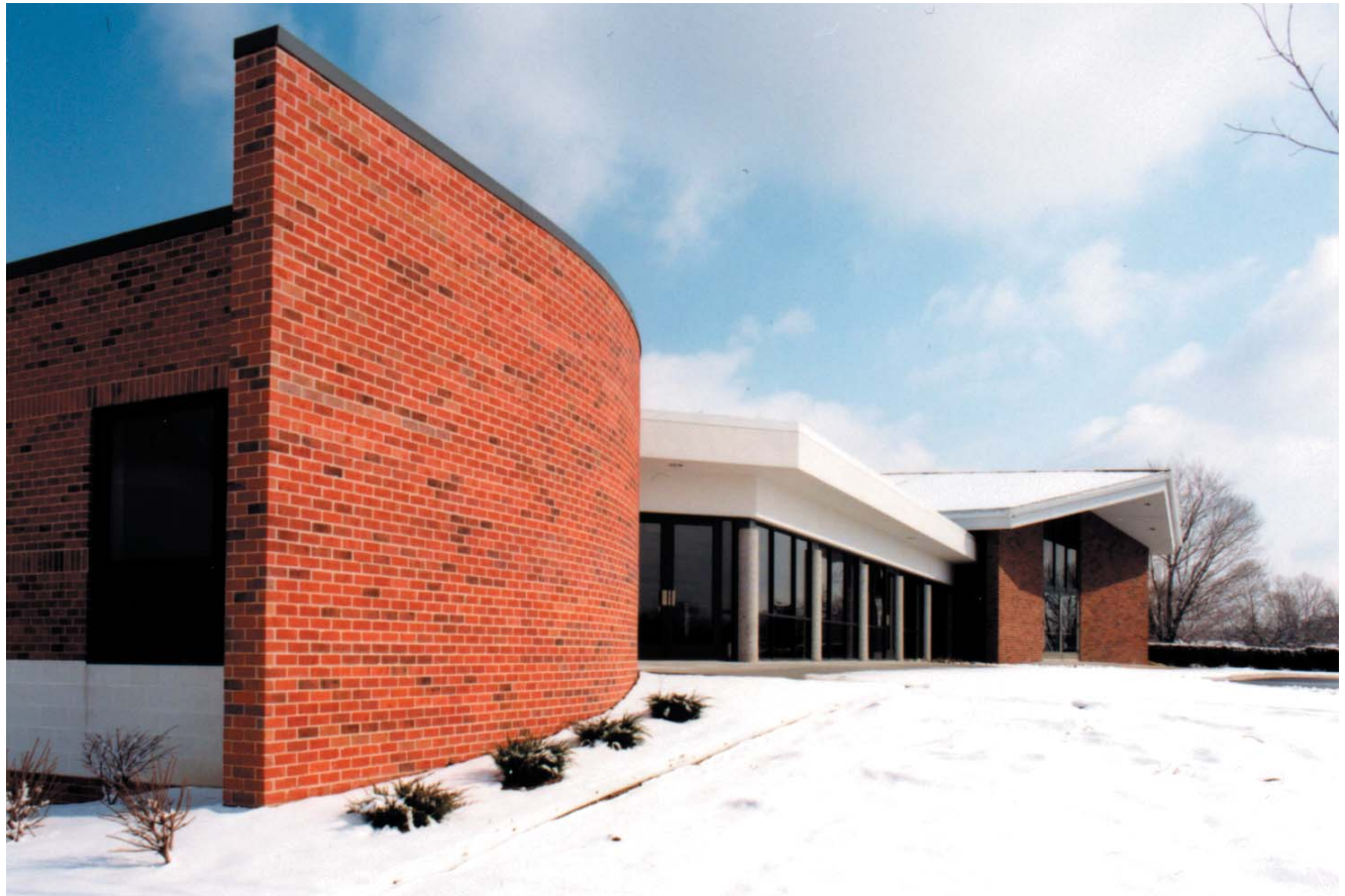
after: curved wall at exterior
