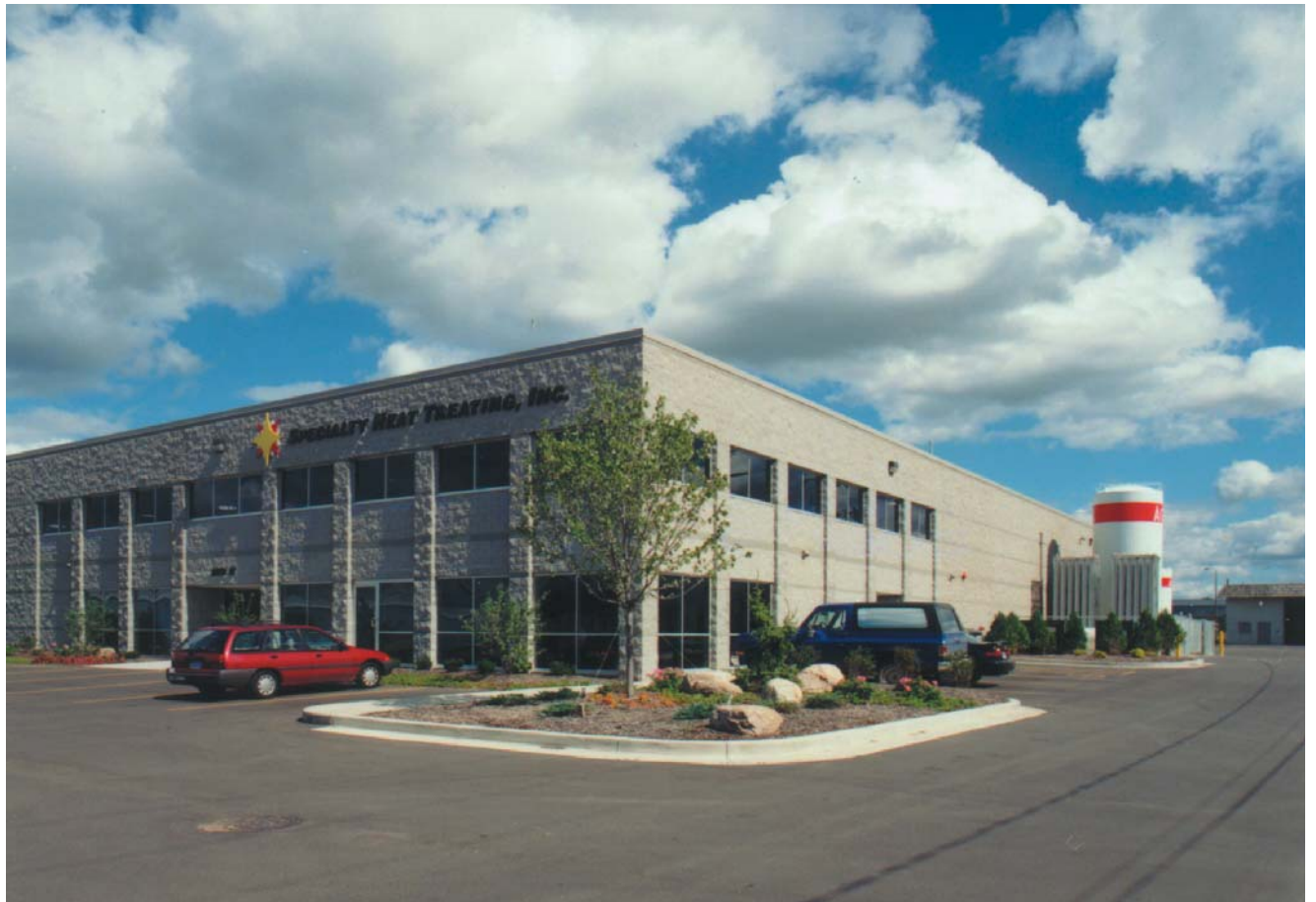
integration of office and industrial functions at exterior
