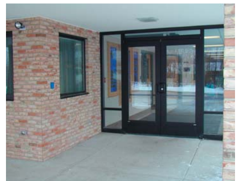
interior view of new entry
