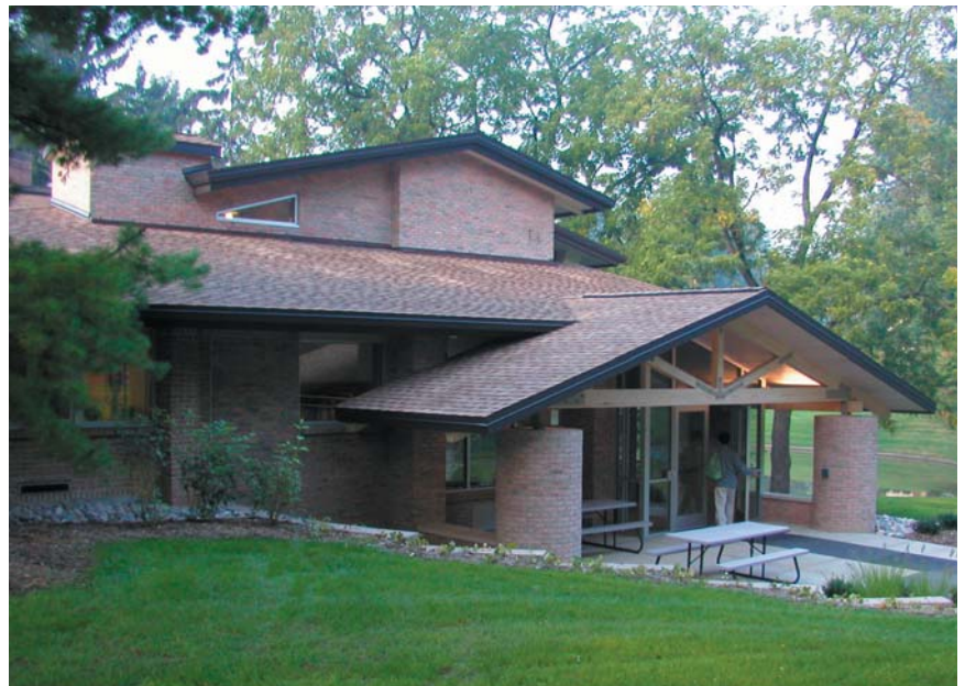
new northwest entry - exterior
